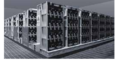
Livestock battery chamber
